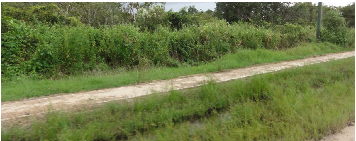
Image 10 – Concrete walking tracks in our town
