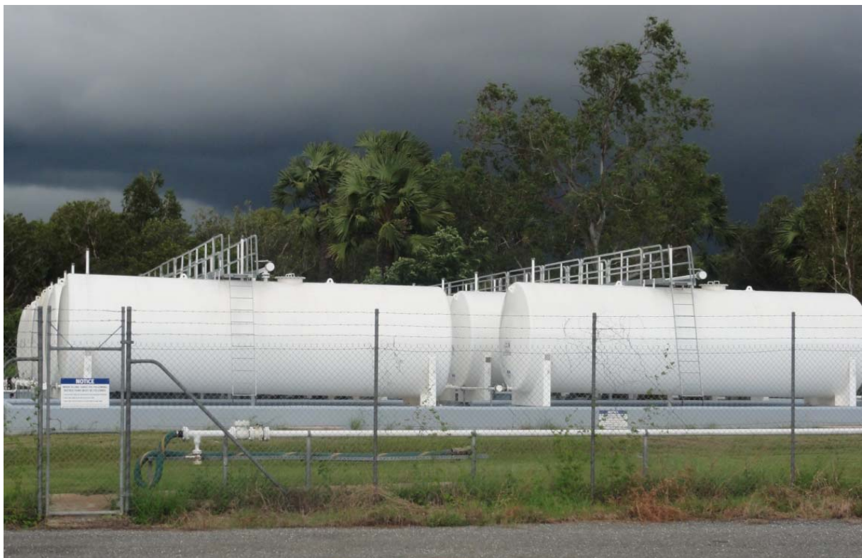
Image 9 – Infrastructure in our town
